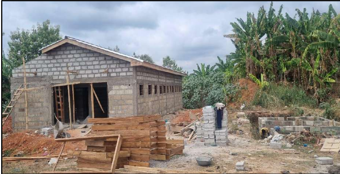
Annex 4: 1 No. 16-Seater water-closet toilet facility – Adadientem (On-going)
