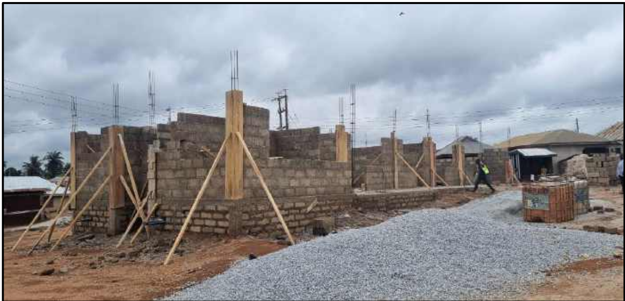
Annex 2: 1 No. 2-Unit KG Block at Ejisu Experimental Basic School - Ejisu (On-going)
