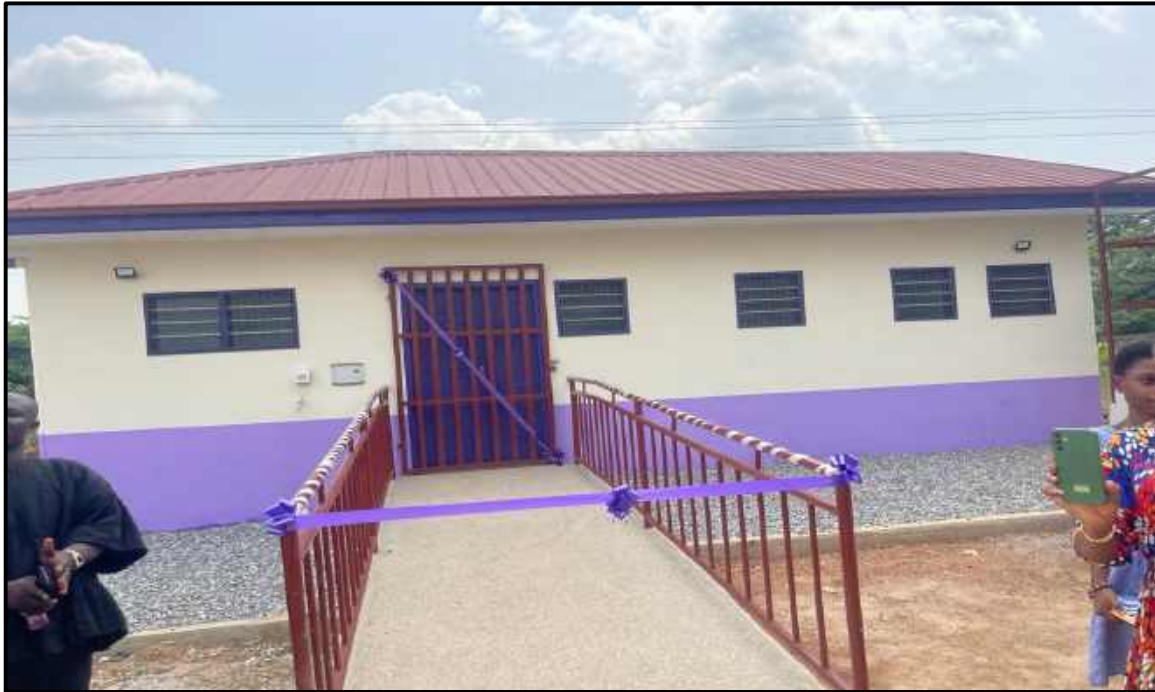
Annex 4: 1 No. 16-Seater water-closet toilet facility – Adadientem (On-going)
